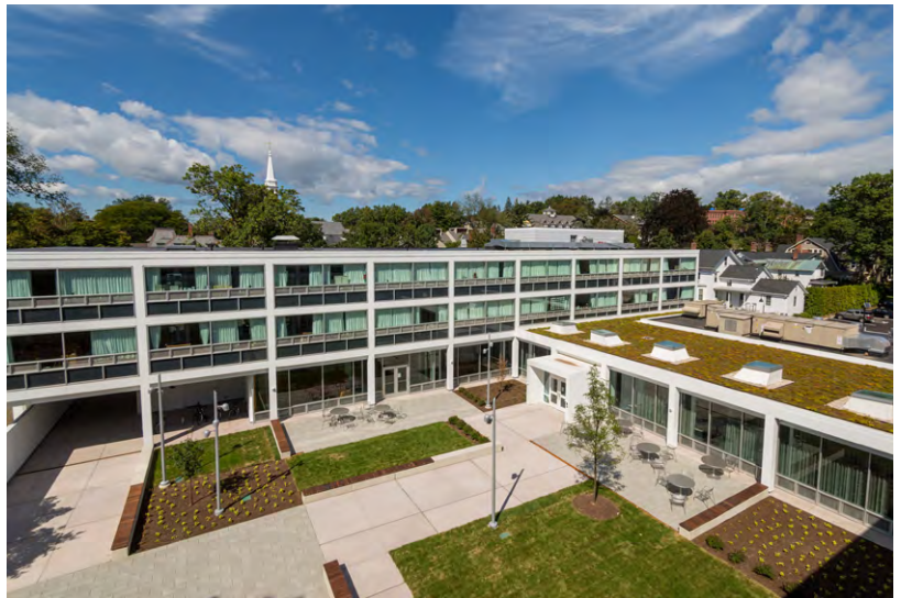
The refurbished Ziskind showing the sedum roof above the dining hall and the redesigned courtyard
