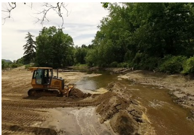
A bulldozer moving sediment for redistribution in Paradise Pond. Approximately 600 cubic yards of sediment was moved to in front of the dam, ready for sluicing.
